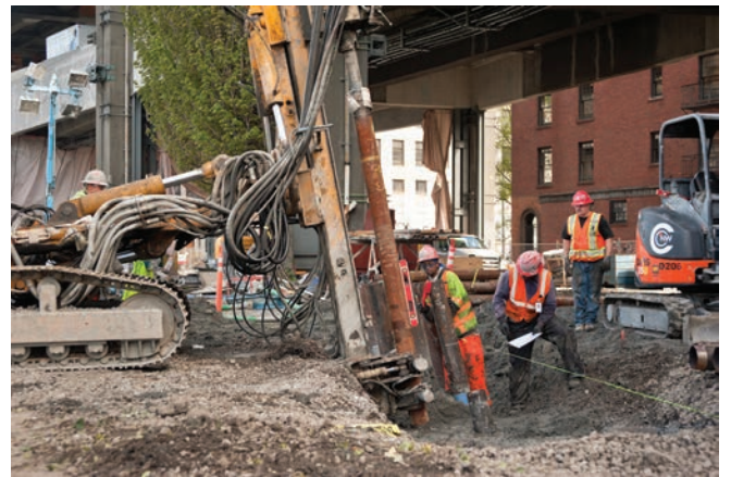
In 2012, crews installed steel micropiles underground to protect the Alaskan Way Viaduct from possible settlement during tunneling.
